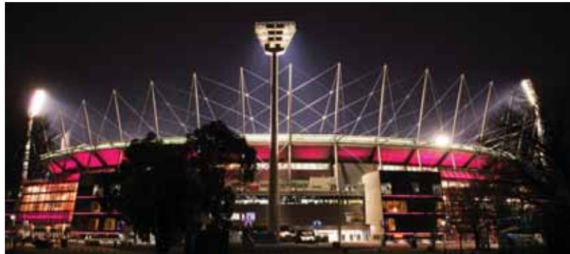
Exterior lighting at the MCG enables sporting codes to theme the stadium in team colours.
